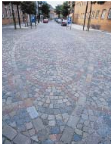
Intricate paving detailing. Note the lack of grade separation between the sidewalk and the street. Image: Hamilton 2000
