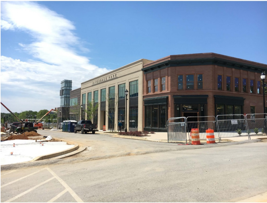
Picture: Riverdale Park Station construction progress: June 2017
