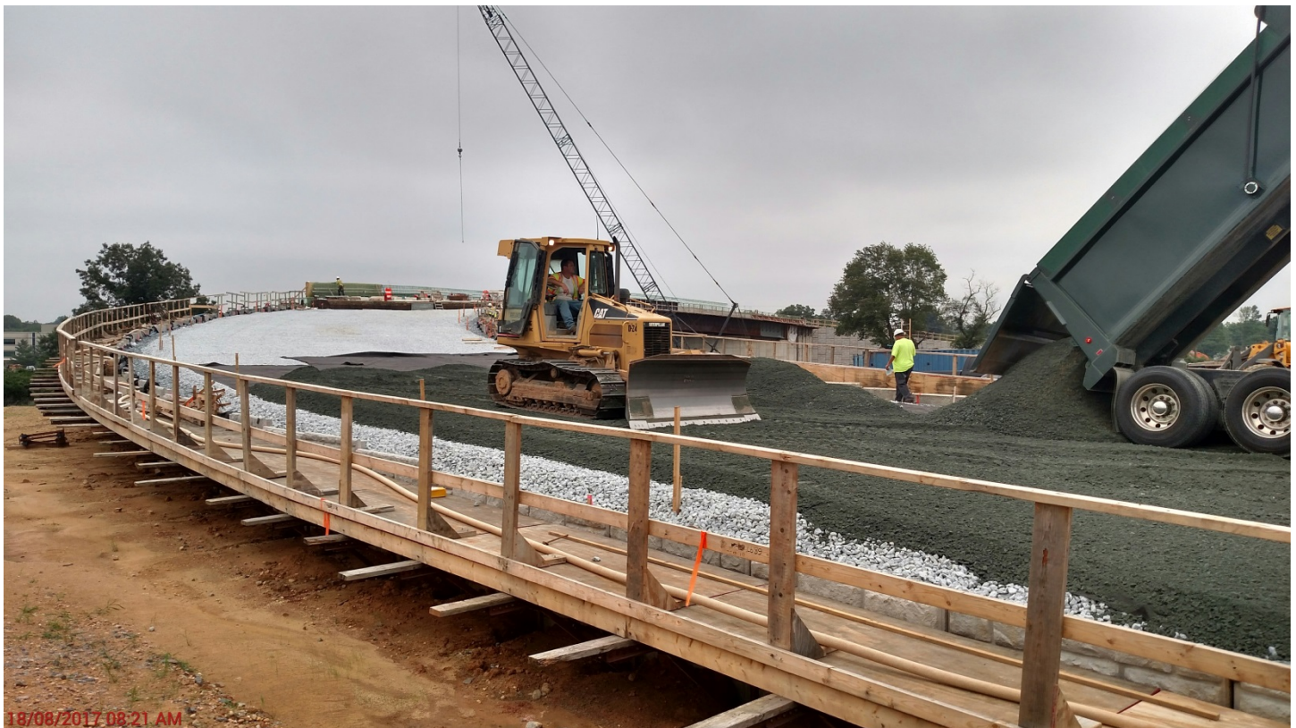
Picture: Future CSX Bridge – Looking East – August 18, 2017
