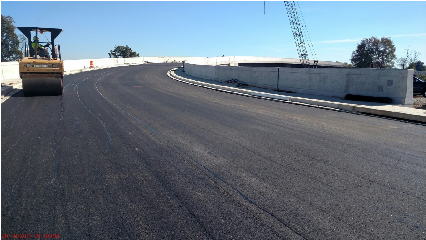
Picture Below: Paved CSX Bridge – Looking East
