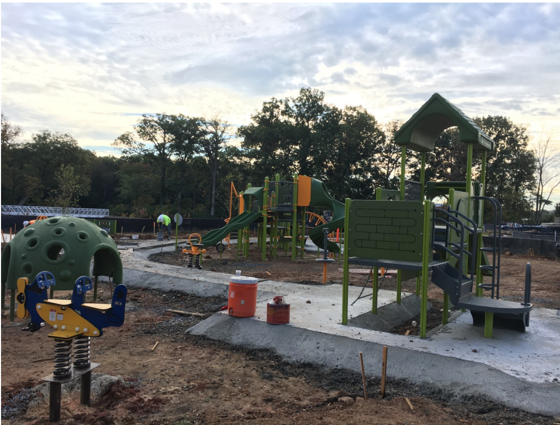
Picture Below: Playground Construction
