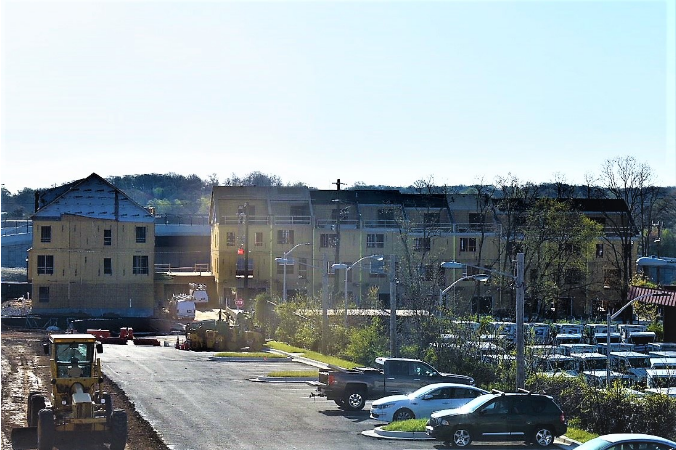
Picture Below: Townhome Construction Progress as of 4/27/2018
