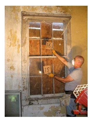
Window "A" from interior, north elevation, showing damaged and missing muntins in both sash which will be recreated.
