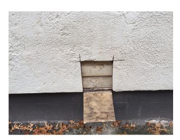
East elevation. Portion of stucco removed to show original drop siding underneath, which will be restored.
